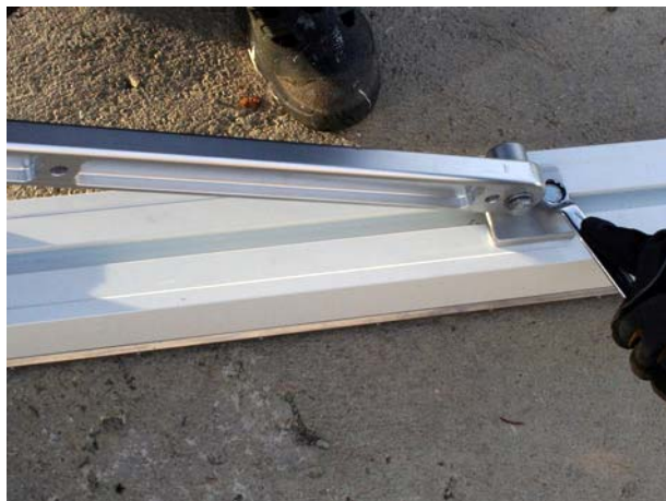
d. Tighten the upper bolt loosely.
